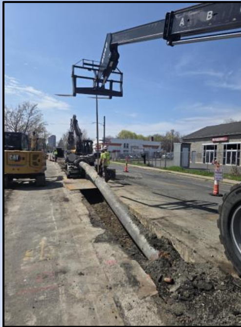
Bypass Piping Setup (Project: Sewer & House Connection Rehabilitation in North Meadows Area)
