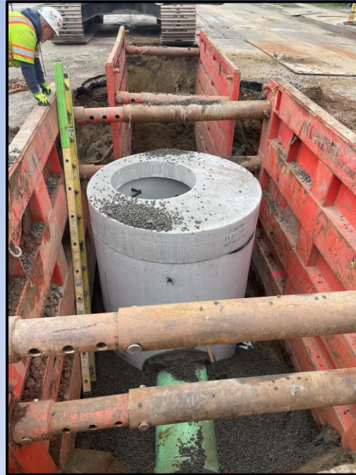
Storm Manhole Installation (Project: Westland Street Area Expedited Sewer Separation)
