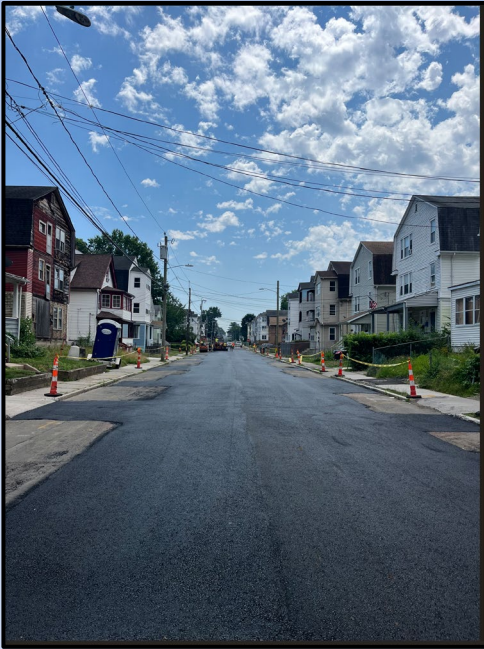
Road Restoration (Project: Westland Street Area Expedited Sewer Separation)
