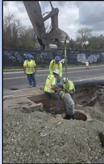
Bypass Piping Setup (Project: Sewer & House Connection Rehabilitation in North Meadows Area)
