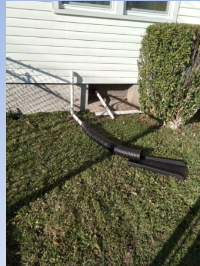
Sump pump discharge to lawn
