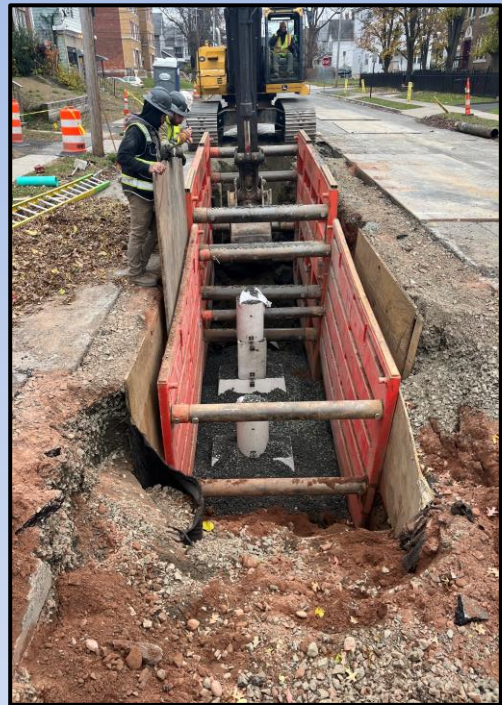
New Storm Drain Installation (Project: Westland Street Area Expedited Sewer Separation)
