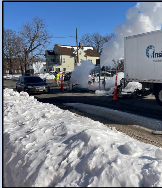
Sewer Lining (Project: Sewer & House Connection Rehabilitation in Gully Brook Area)
