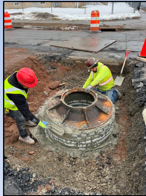
Manhole Install (Project: Westland Street Area (CFQ-13))
