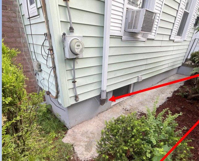
Project: Woodstock and Branford Streets Expedited Sewer Separation
