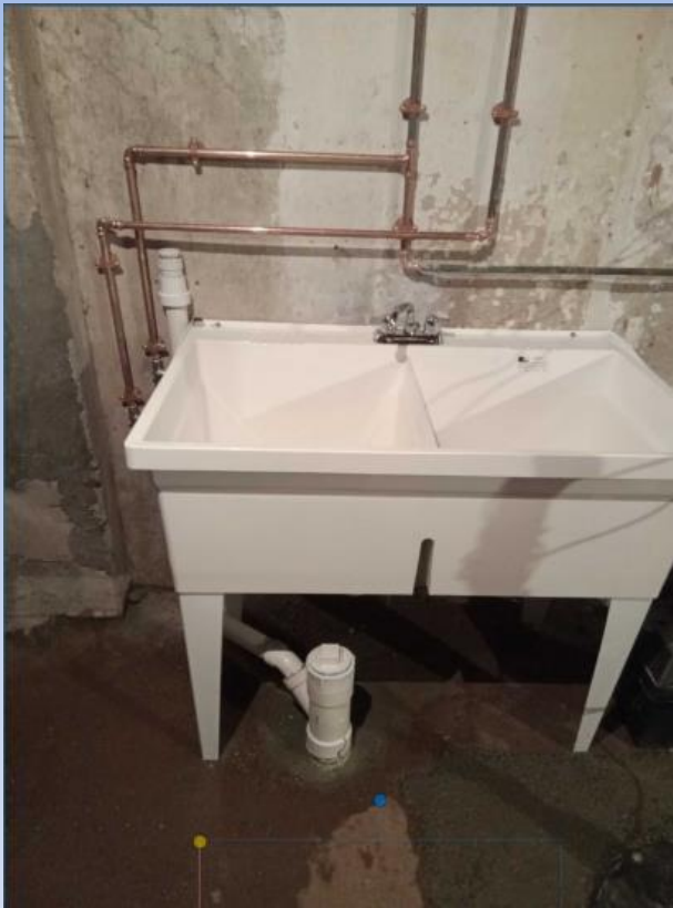
New double bay plastic sink and drain piping (new check valve also installed not in photo)
