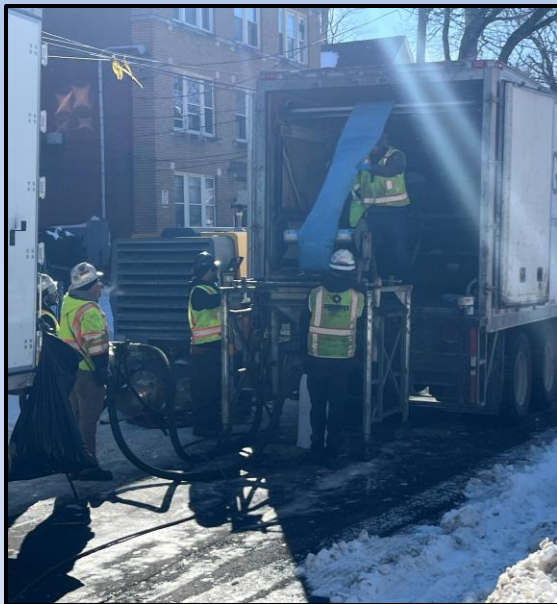
Sewer Lining (Project: Sewer & House Connection Rehabilitation in Gully Brook Area)
