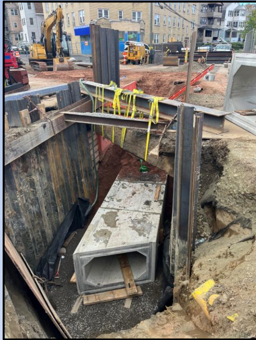
New Storm Drain Installation (Project: Westland Street Area Expedited Sewer Separation)
