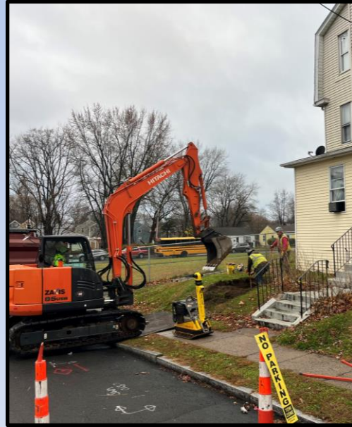
Lateral Repair (Project: Sewer & House Connection Rehabilitation in Gully Brook Area)
