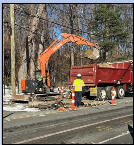
Lateral Repair (Project: Sewer & House Connection Rehabilitation in Gully Brook Area)
