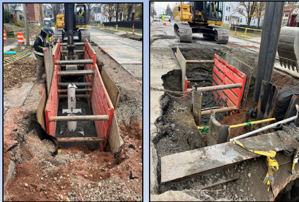
New Storm Drain Installation (Project: Westland Street Area Expedited Sewer Separation)
