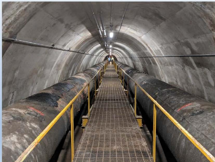
Photo: Steel Mains within Saville Dam Gatehouse
