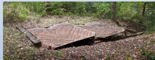
Photo: Rotted Wooden Protective Deck at Weir
