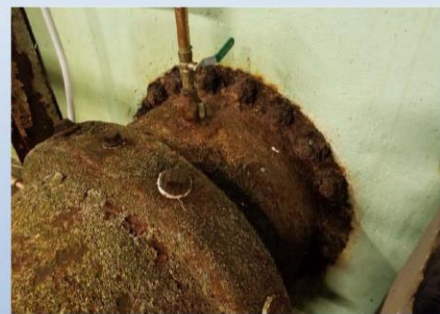
Photo: Corroded Pipe
