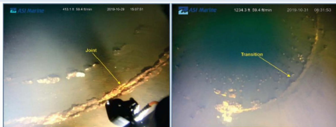
Figure 19: Image of joint at Station 03+41 (left); Image of transition at Station 12+17 (right)
