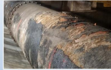
Photo: Damaged Exterior Coating
