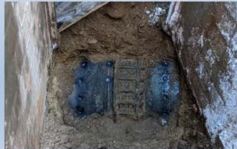
Photo: Exposed Dresser Coupling
