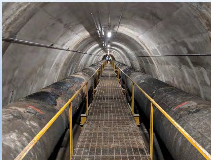
Photo: Steel Mains within Saville Dam Gatehouse
