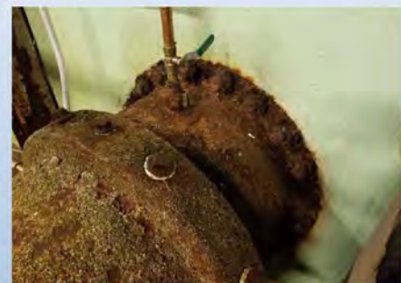
Photo: Corroded Pipe
