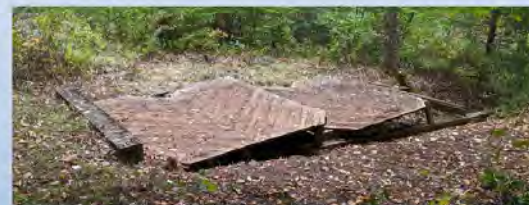
Photo: Rotted Wooden Protective Deck at Weir
