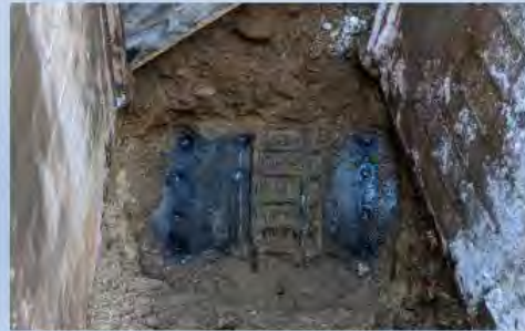
Photo: Exposed Dresser Coupling
