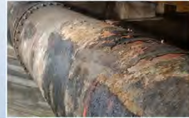
Photo: Damaged Exterior Coating
