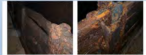
Photos: Baffle deterioration
