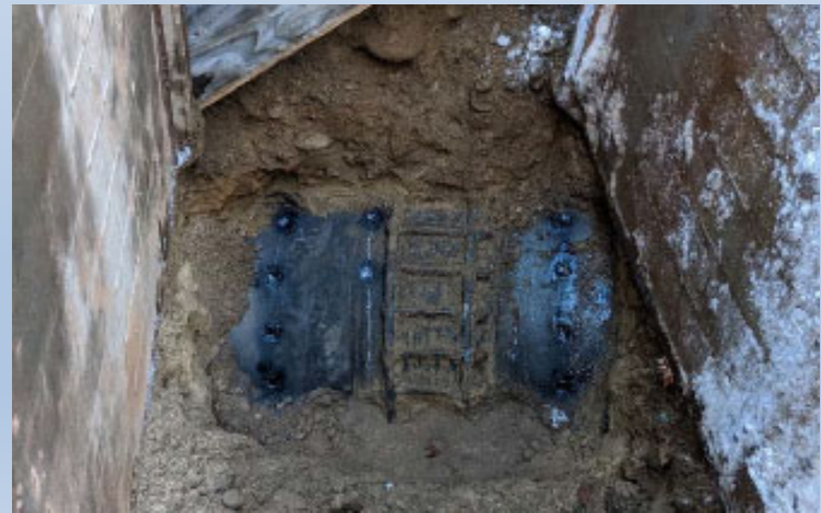
Photo: Exposed Dresser Coupling
