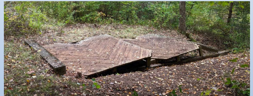
Photo: Rotted Wooden Protective Deck at Weir
