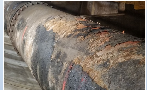
Photo: Damaged Exterior Coating
