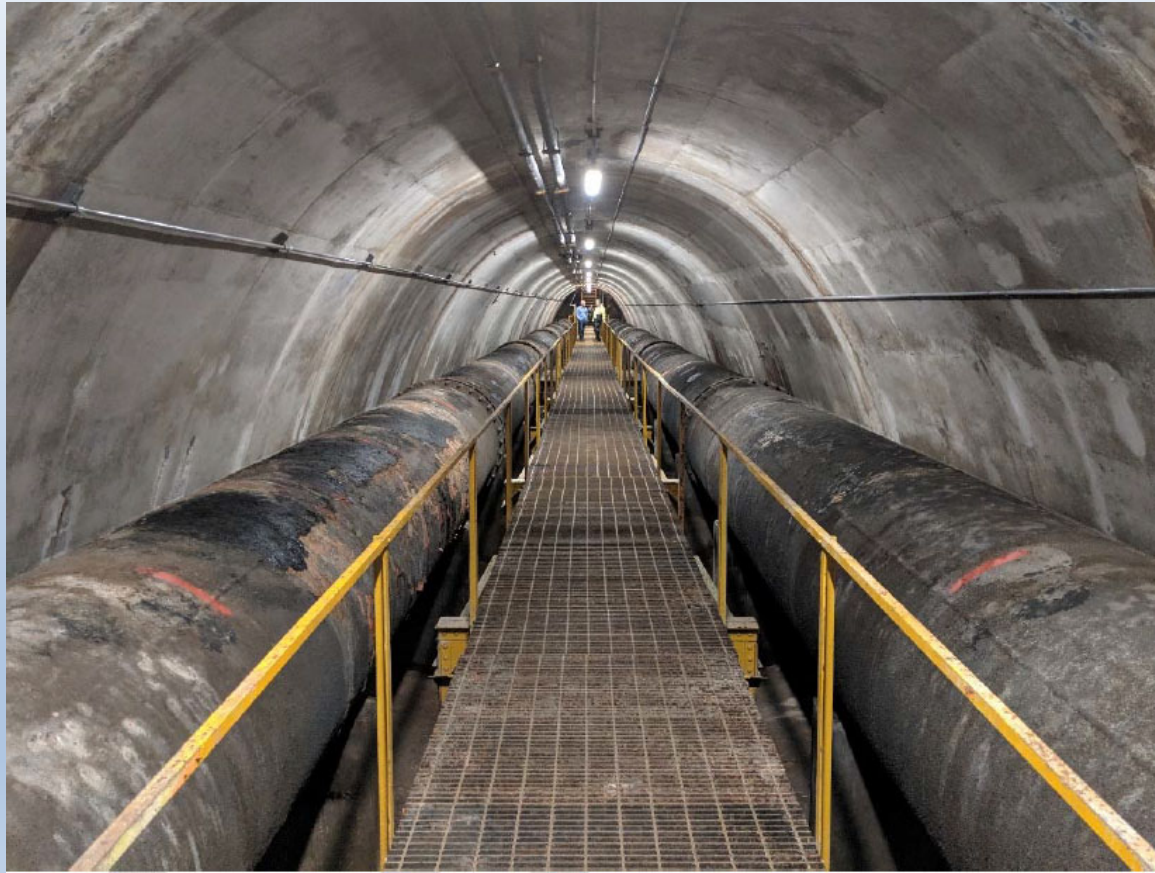
Photo: Steel Mains within Saville Dam Gatehouse
