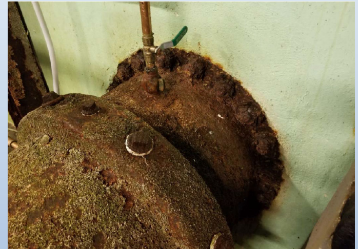
Photo: Corroded Pipe
