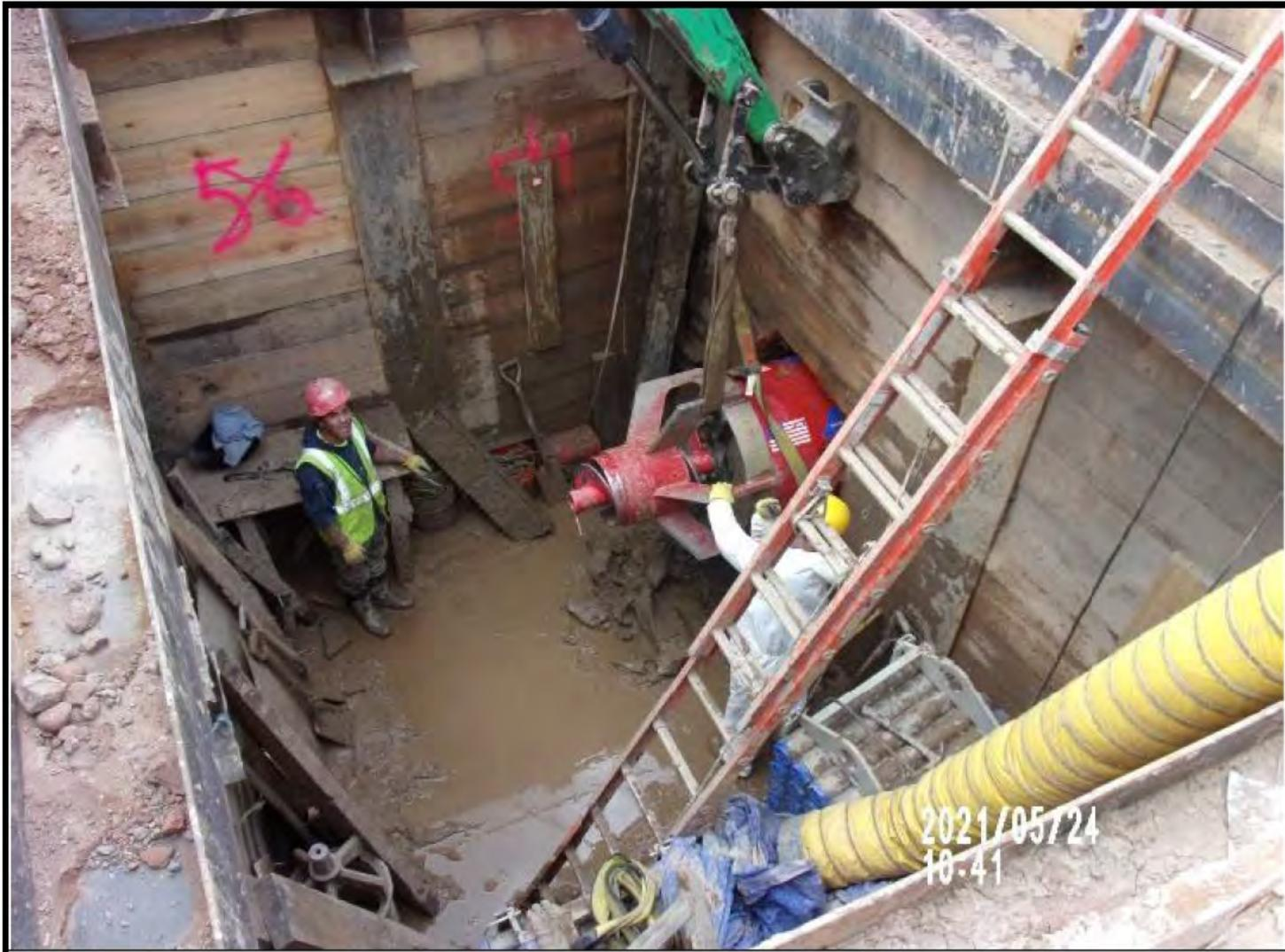
Contract 5 – Junction manhole at DS-2. Microtunnel pipe connected to reinforced concrete structure – Hartford.
