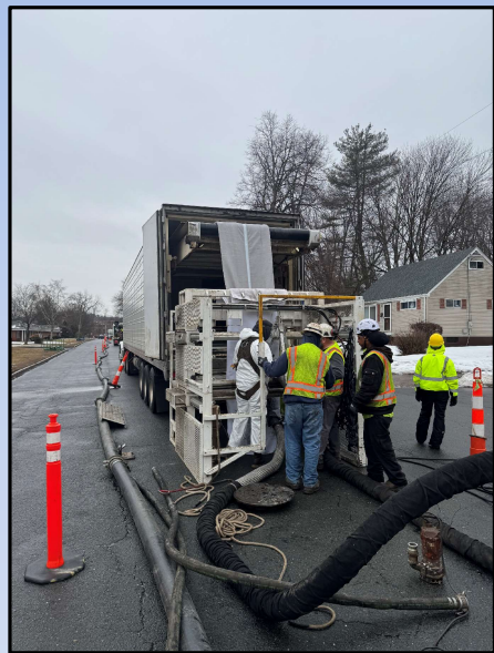
Sewer Main Rehabilitation (Project: Sewer & House Connection Rehabilitation in Gully Brook Area)
