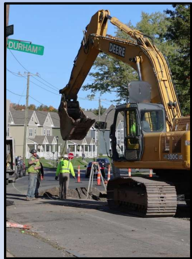
Point repair (Project: Sewer & House Connection Rehabilitation in North Branch Park River Area)
