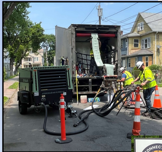
Mainline CIPP (Project: Gully Brook Area Sewer & Lateral Rehabilitation/Repair)
