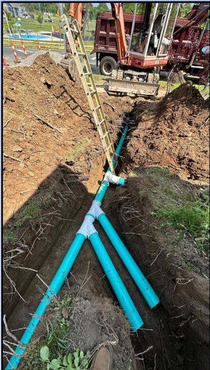
New Storm Lateral (Project: Woodstock and Branford Streets Expedited Sewer Separation)
