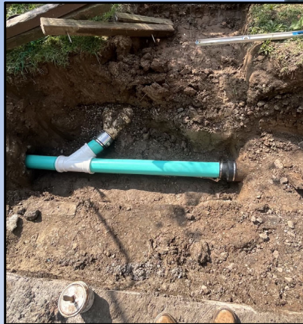
Lateral Repair (Project: Sewer & House Connection Rehabilitation in North Meadows Area)
