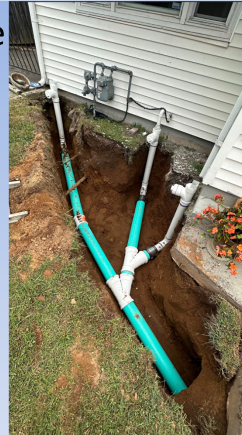
Project: Woodstock and Branford Streets Expedited Sewer Separation
