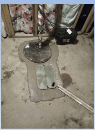
New sump pump (with battery backup) and new BWV inside irrigation style box
