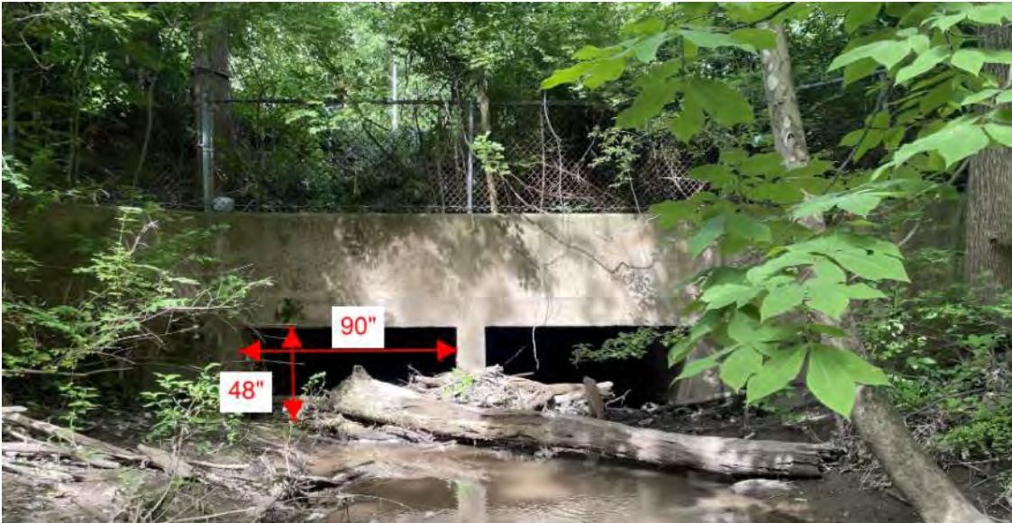
Looking downstream, toward Mark Twain Drive Field Visit June 3, 2024
