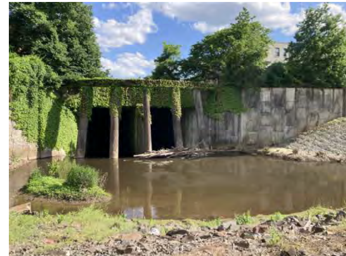
Debris dam after cleaning, May 28, 2024
