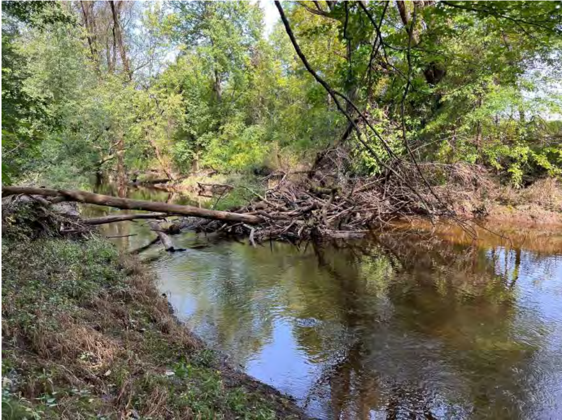
Photo 42: Downed trees in Segment 4, trees creating debris dam (see Figure 3-4, TD-22).
