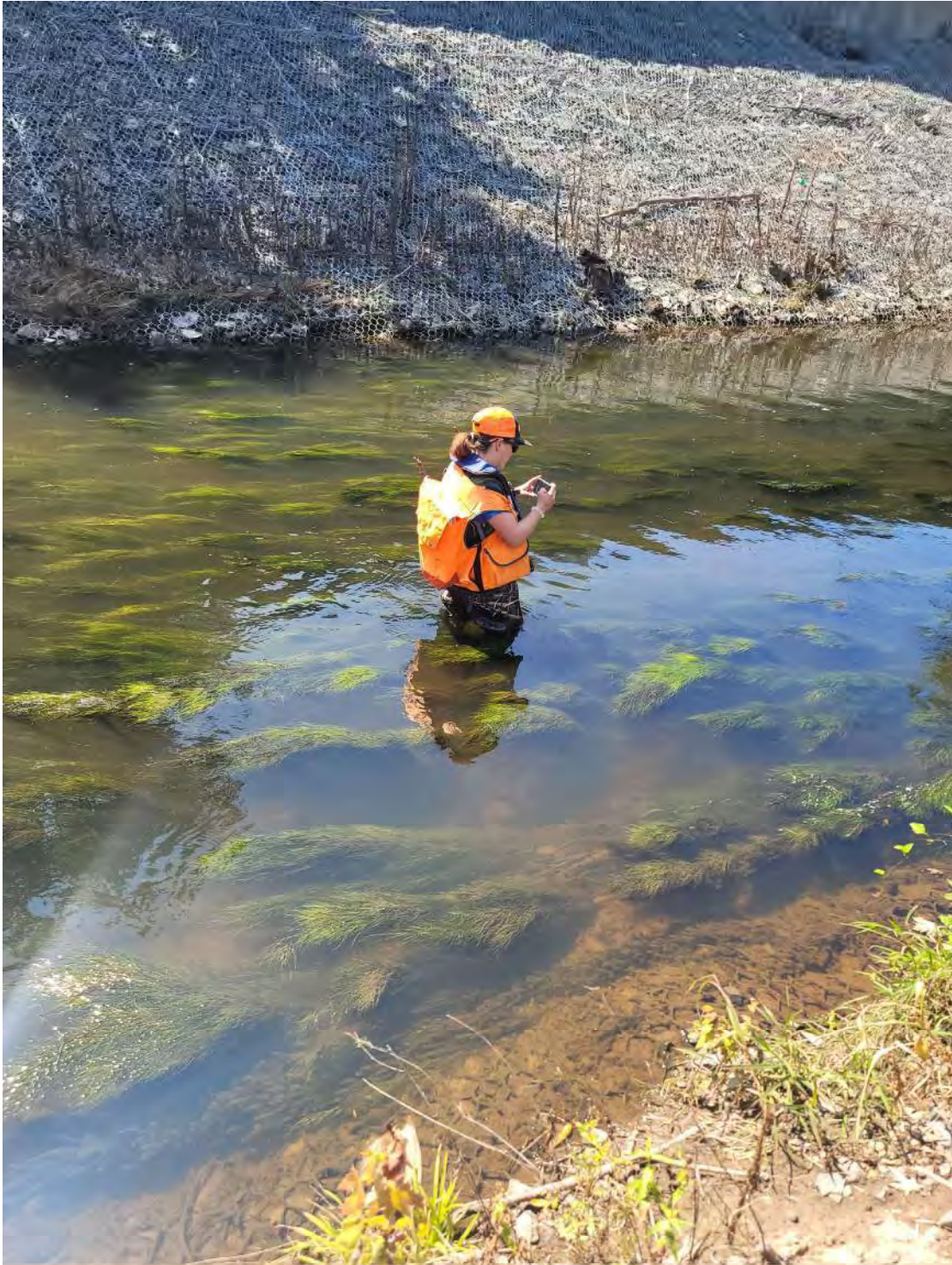
Photo 5: Segment 1 with chain link fence over rip rap armor.
