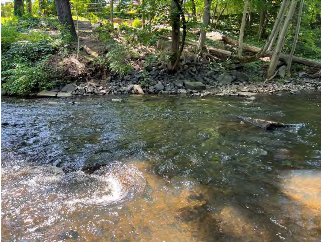
Photo 6: Small-gauge rip rap/naturalized rock channel with areas of riffles and runs and vegetated, gently sloping banks (Segment 1).
