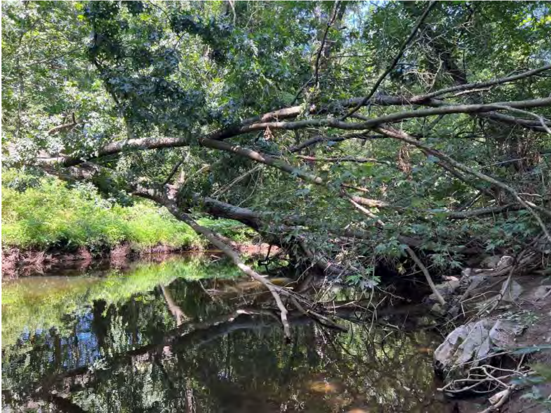
Photo 10: Debris dam behind 21 Woodland Street within Segment 1 (See Figure 3-1, TD-3).
