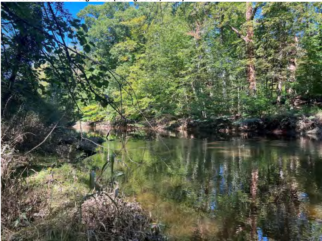
Photo 31: Example of near vertical banks on the opposite bank in Segment 3.
