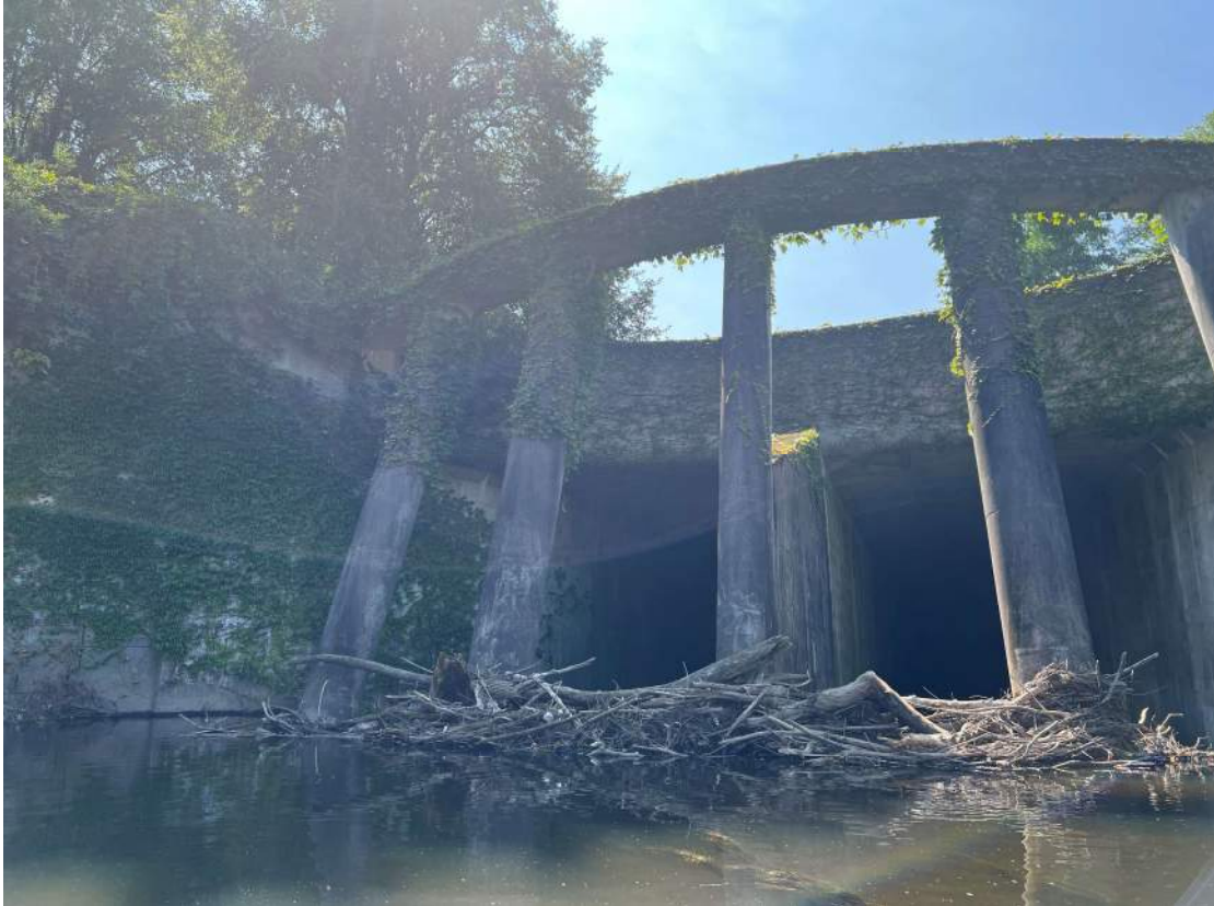
Photo 1: Debris dam at start of Segment 1, Park River Conduit (See Figure 3-1, TD-1).
