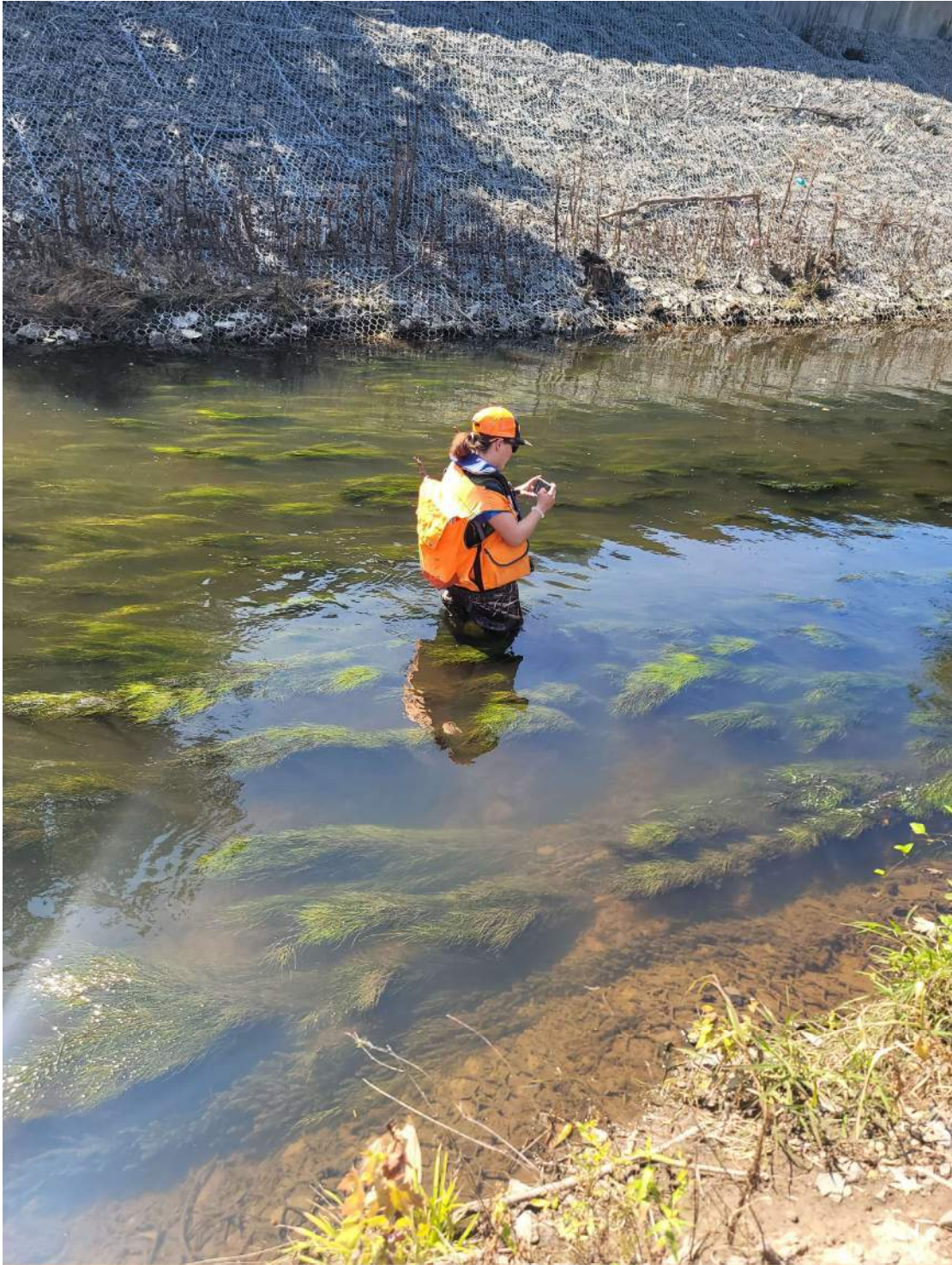
Photo 5: Segment 1 with chain link fence over rip rap armoring.
