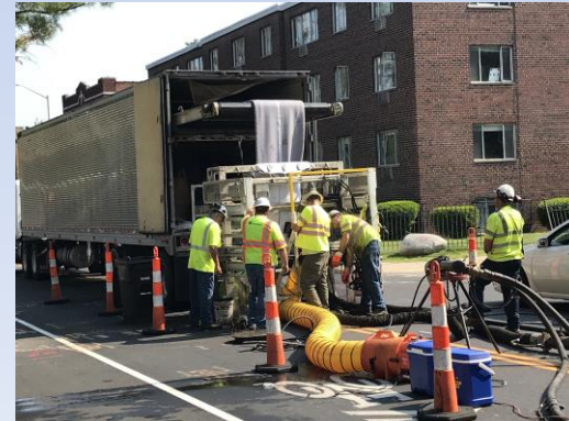
Sewer Main Lining
