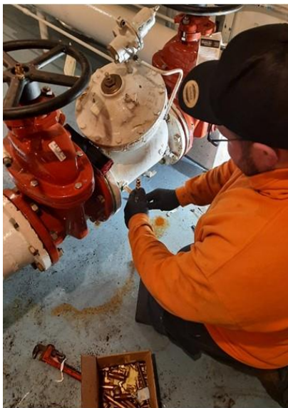
Pressure Reducing Valve - Farmsted SPS
