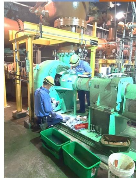
HWPCF RAS Pump - Aligning pump and motor
