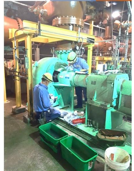
HWPCF RAS Pump - Aligning pump and motor
