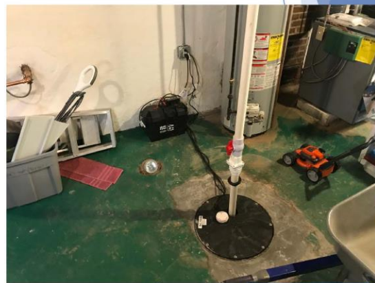
INSTALLED SUMP PUMP WITH BATTERY BACK UP
