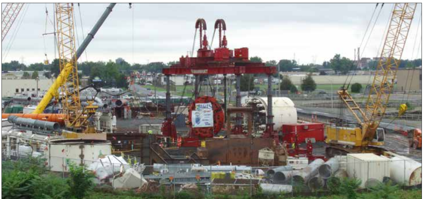
The cutterhead and gantry at the launch shaft
