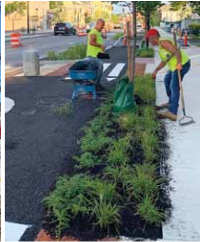
Mulch placement at tree pits
