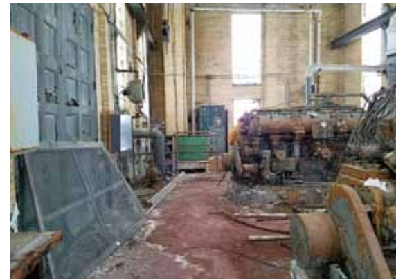
Pump station pre-restoration
