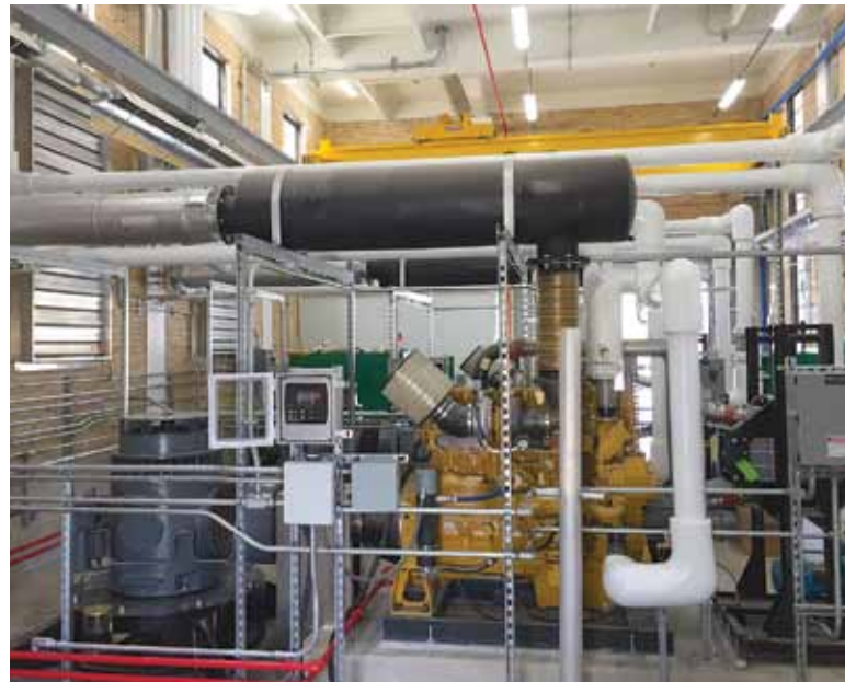
Lowell's restored flood pump station
