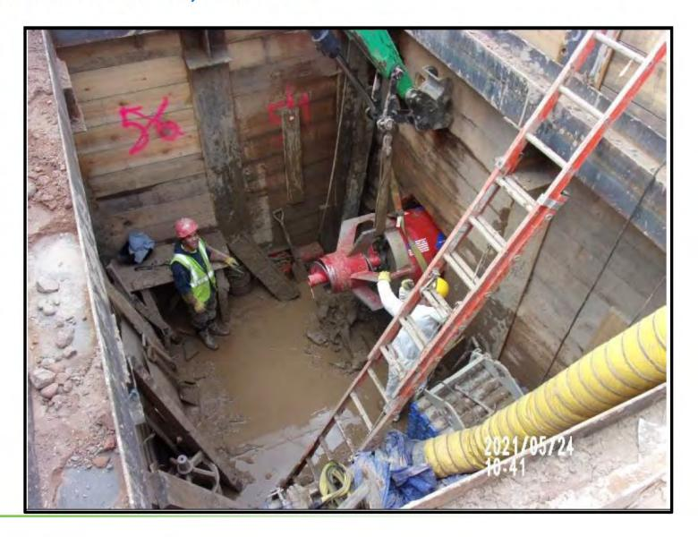
Contract 5 – Junction manhole at DS-2. Microtunnel pipe connected to reinforced concrete structure – Hartford.
