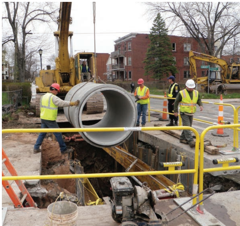
During a sewer separation project in Hartford, workers add a second pipe in the street to serve as a sanitary sewer.
