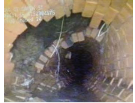
Figure 4 Pipe Collapse
