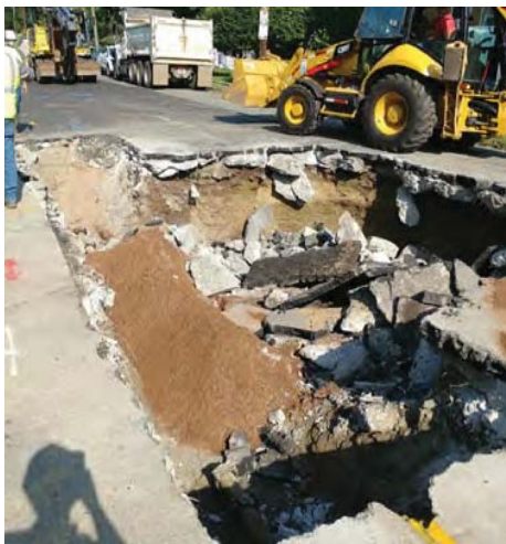
Figure 3 Capen Street Sinkhole from Pipe Failure
