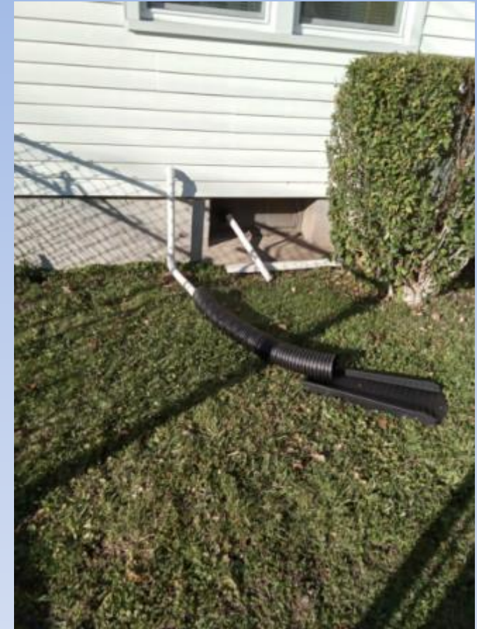
Sump pump discharge to lawn
