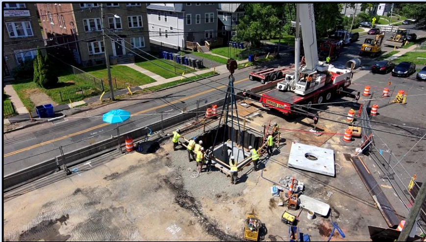
New Storm Drain Installation (Project: Westland Street Area Expedited Sewer Separation)
