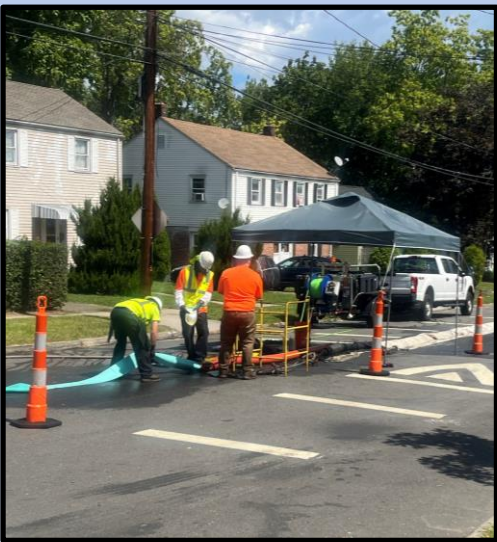
Lateral Lining (Project: Sewer & House Connection Rehabilitation in Gully Brook Area)
