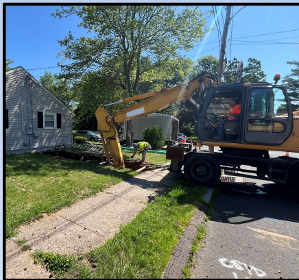
Lateral repair (Project: Sewer & House Connection Rehabilitation in Gully Brook Area)
