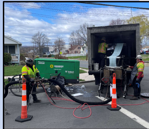
Mainline CIPP (Project: Sewer & House Connection Rehabilitation in North Branch Park River Area)
